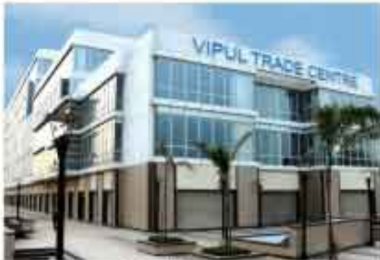
Vipul Trade Centre, Gurgaon
